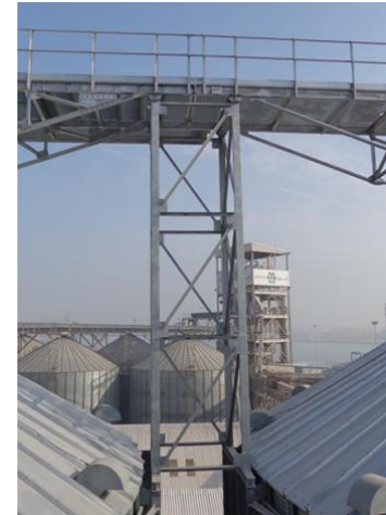
Fig. 2: Detail of catwalks directly supported over silos
