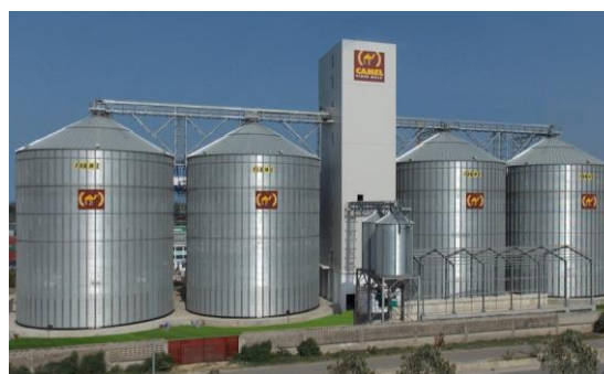
Fig. 1: 24.000 T Plant in Dar Es Salaam, Tanzania
